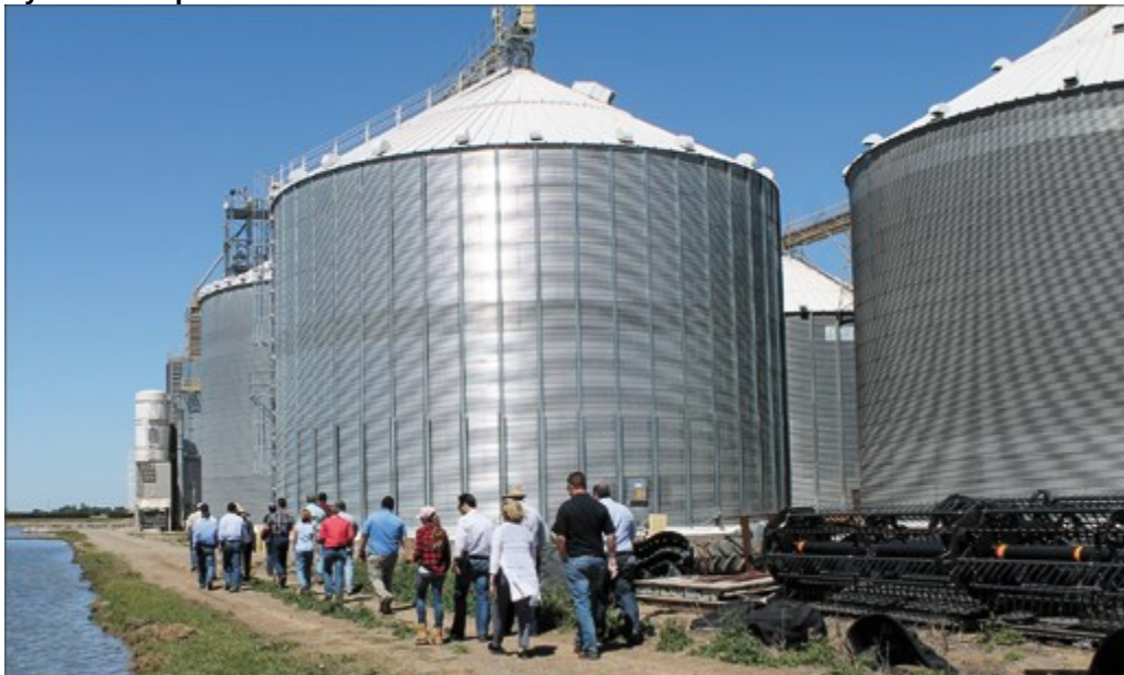
The rice bins shown here might have to be raised as much as 20 feet off the ground to comply with flood zoning rules. Photo/Kate Campbell
